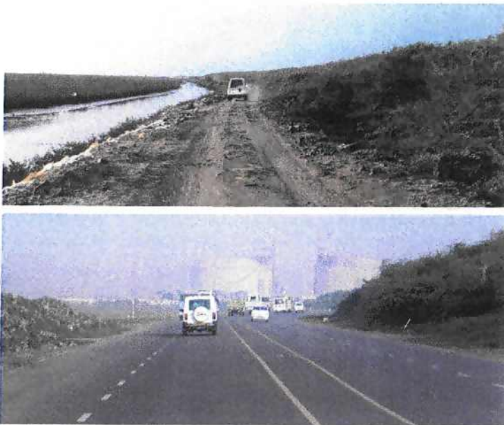
Figure 12 Initial dirt road along the coast and completed access road to Hazira port
