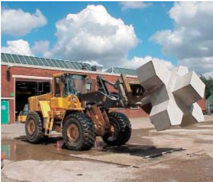
Figure 14. A forklift was the most suitable equipment for handling the Xbloc.
