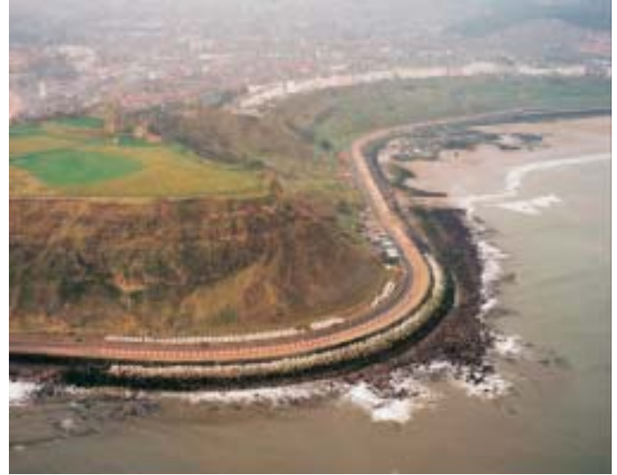
Figure 2. Concrete armour units are generally applied in breakwaters (left, Scheveningen, The Netherlands) and shore protections (right, Scarborough, U.K.).
