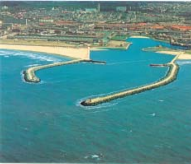
Figure 2. Concrete armour units are generally applied in breakwaters (left, Scheveningen, The Netherlands) and shore protections (right, Scarborough, U.K.).
